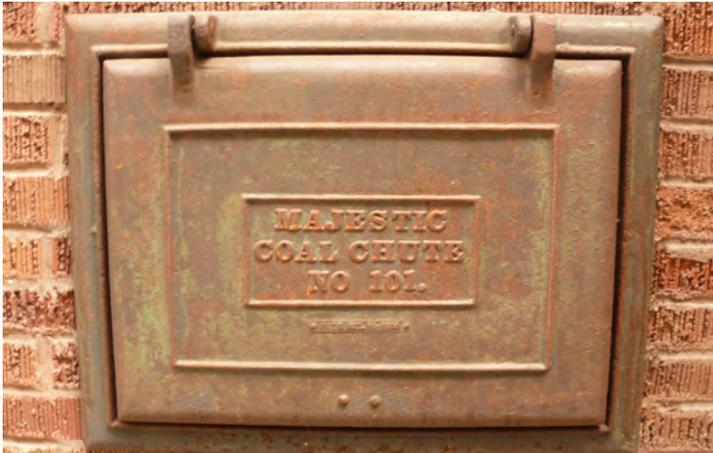
A surviving "coal chute," which had been used to supply a basement coal-burning furnace, which were common through the 1950s.
