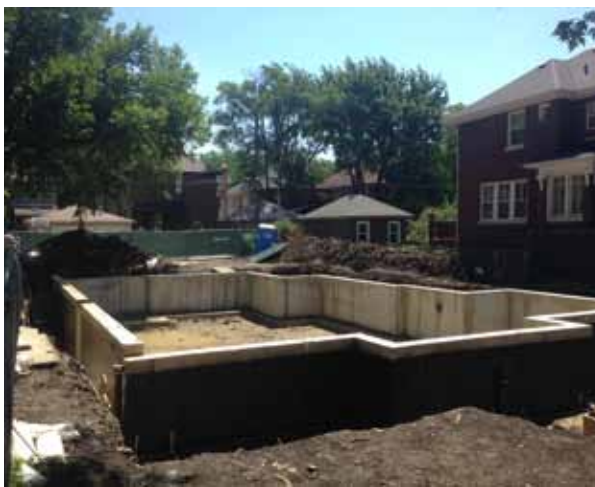
Top: This Chicago Tribune ad from July 1909 illustrates the various styles of “model homes” that potential Ravenswood Manor buyers could choose from. Bottom: The basement excavation for a new residence that replaced one of the original model homes last year.
