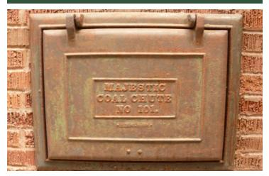
A surviving "coal chute," which had been used to supply a basement coal-burning furnace, which were common through the 1950s.
