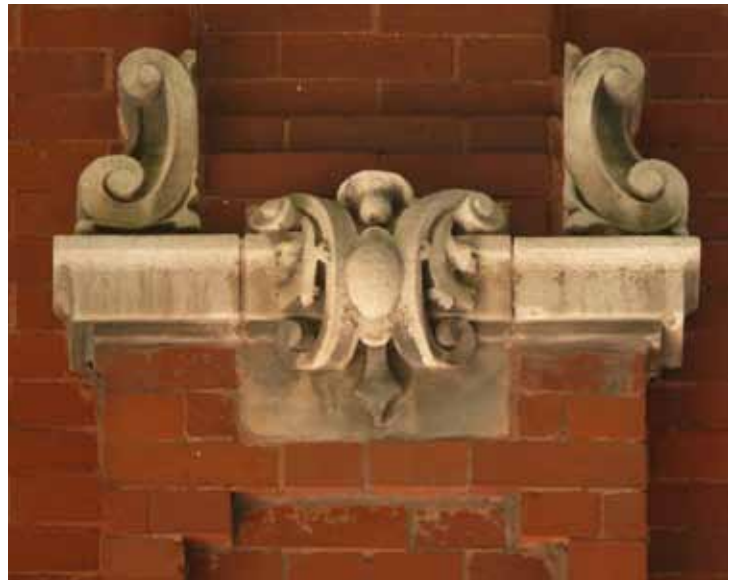
Carved limestone ornament, McDonald-Petrus House, 4444 N. Richmond St. (1909; William Schulze, architect).
