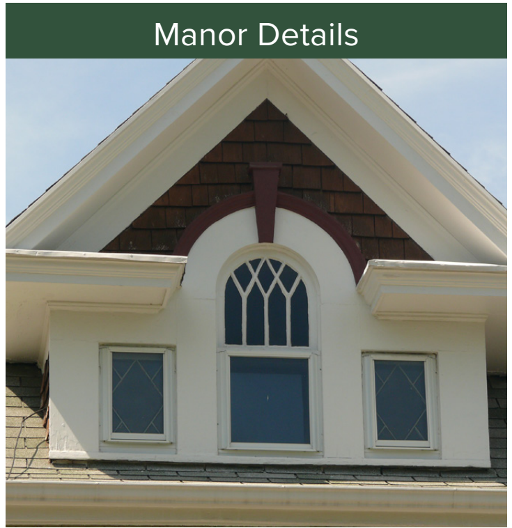
Dormer on early (c.1910) house in the 4500-block of Sacramento Avenue
